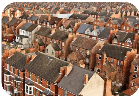
Housing development is supported by the infrastructure
